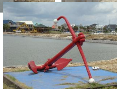
(Marina Construction as of 29-Jun-10)
